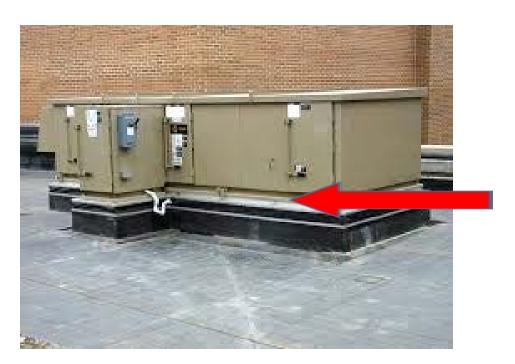
Displaces neoprene and is a continuous gasket bonded between the HVAC unit and curb surfaces to seal against water and weather conditions.
